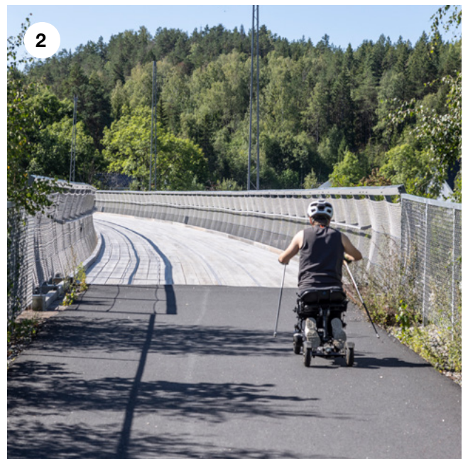
1) DERAILED: The 150-metre-long Hølen viaduct connects the old train route between Kjenn and Sonsveien station to create a continuous footpath. 2) FULL SPEED AHEAD: The railroad tracks have been removed and the bridge itself is now a wooden path that can be used by walkers, cyclists and everyone else with wheels.
