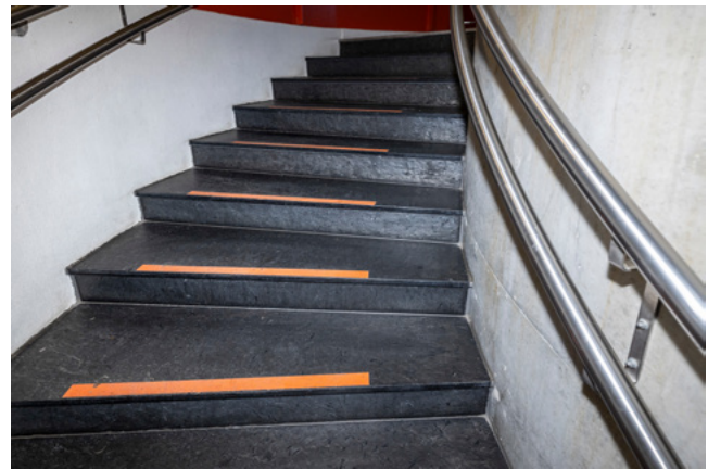
ORANGE CONTRAST: A library user had pointed out that it was difficult to see the black granite steps leading down to the lower level. A single orange contrast stripe solved the problem.
