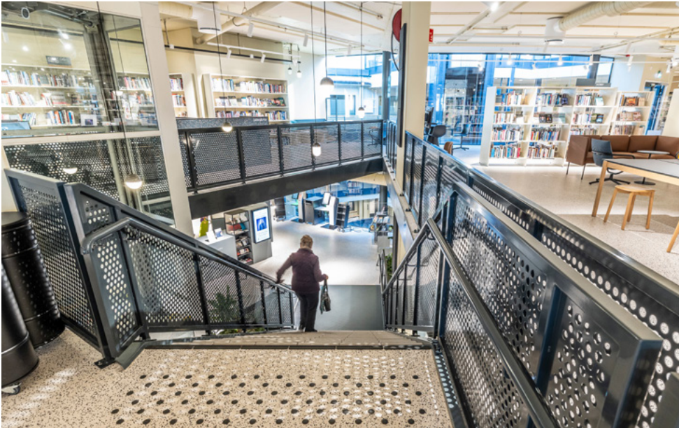
SAFETY FIRST: Handrails, markings and stair nosing make stairs safer to use.
